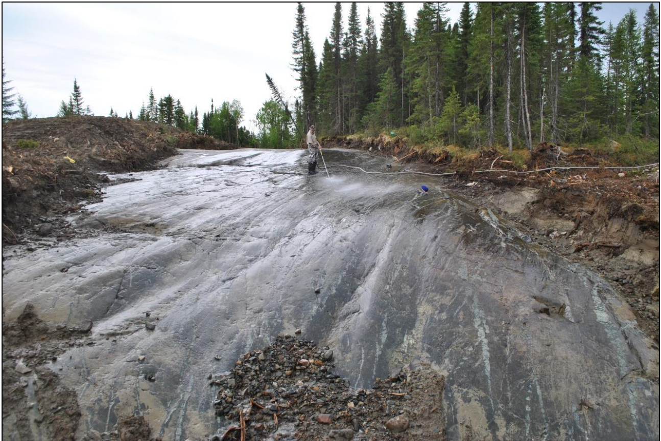
Figure 18: Washing of a stripped area of the South Zone deposit to expose the glaciated bedrock below
